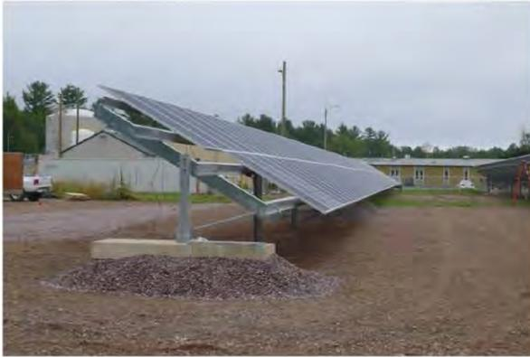
In September 2017, the Marquette Board of Light & Power completed a 0.15 MW(DC) solar facility, using 480 individual 320 watt solar panels.
