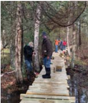
VOLUNTEERS CONSTRUCTING BOARDWALKS AT WEST SIDE TRAILS
