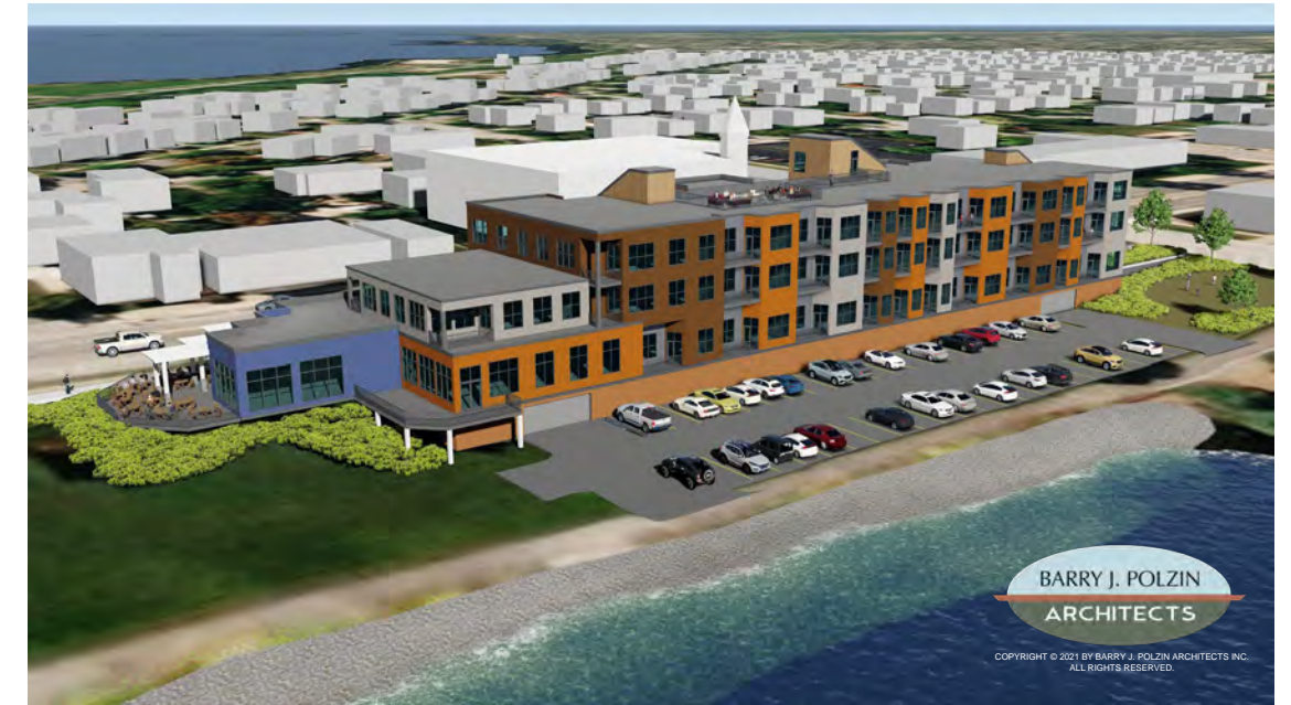
AERIAL VIEW OF NORTH FACADE FROM WATER
