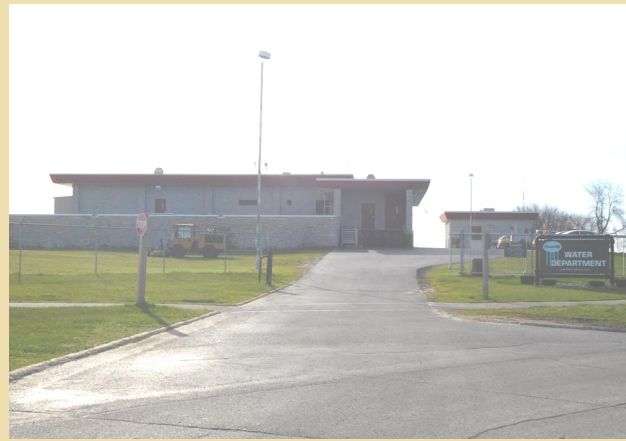
WATER TREATMENT PLANT
