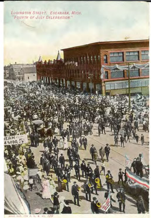
Image 2-3: Masonic Building and Bank, Escanaba circa 1900.
