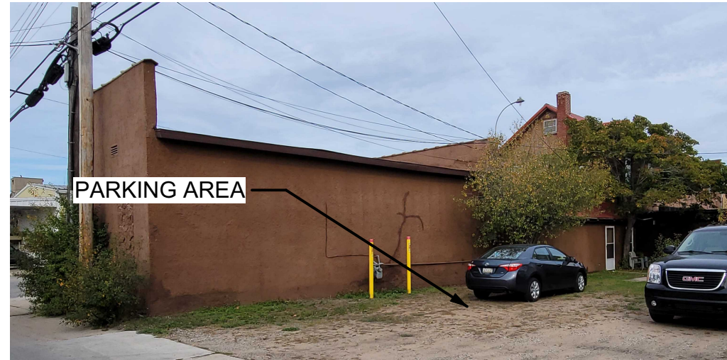
2 REAR AND SIDE (SOUTH) BUILDING VIEW Scale: N.T.S.
