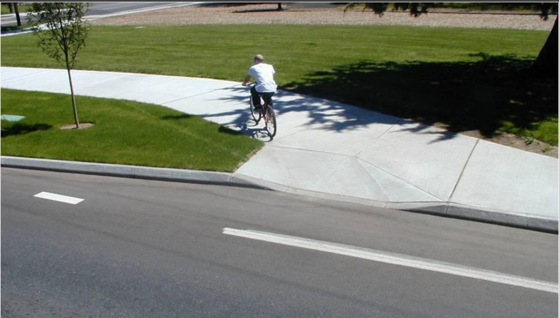
Bicyclist takes exit ramp
