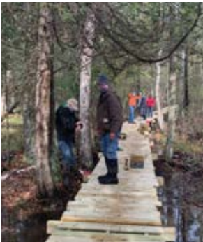
VOLUNTEERS CONSTRUCTING BOARDWALKS AT WEST SIDE TRAILS
