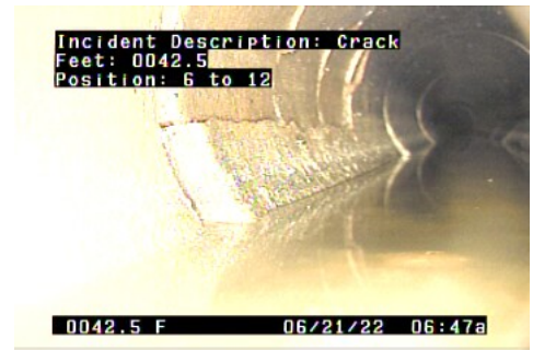
C - Crack @ 42.5 ft.
