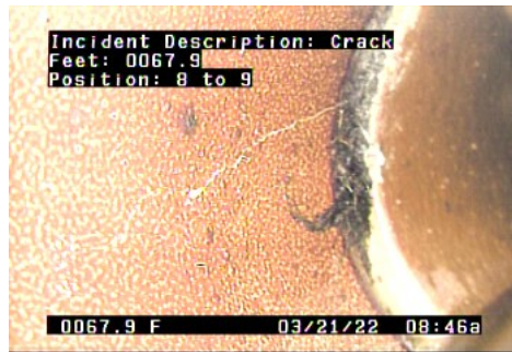
C - Crack @ 67.9 ft.
