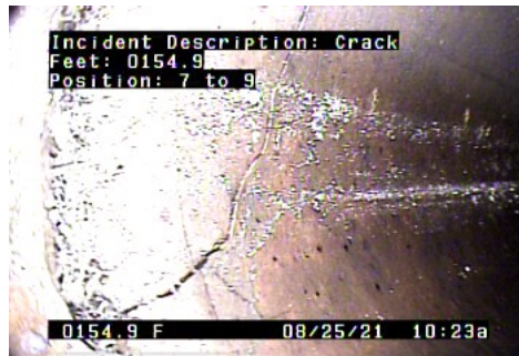
C - Crack @ 154.9 ft.
