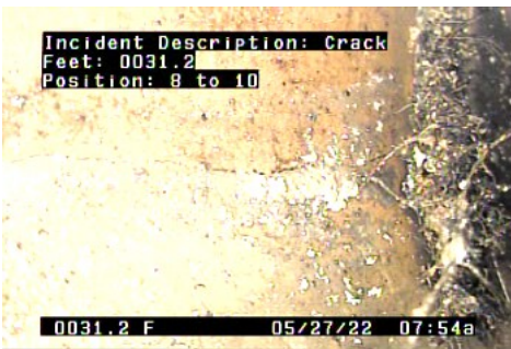
C - Crack @ 31.2 ft.
