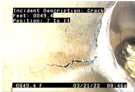
C - Crack @ 49.4 ft.
