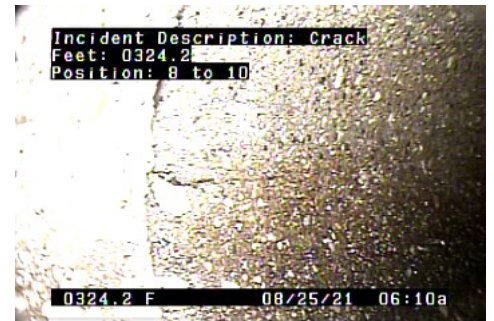
C - Crack @ 324.2 ft.
