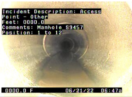
AP - Access Point - Other @ 0.0 ft. Manhole S9457
