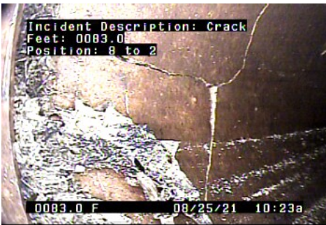
C - Crack @ 83.0 ft.
