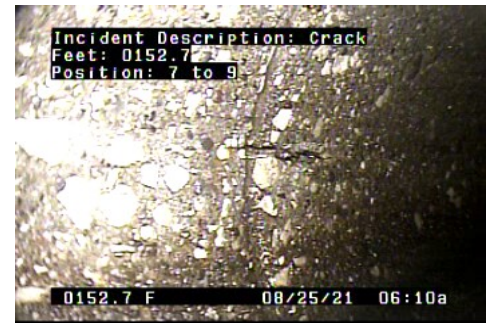
C - Crack @ 152.7 ft.
