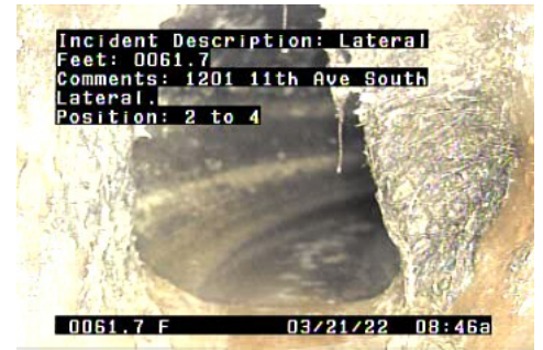
L - Lateral @ 61.7 ft. 1201 11th Ave South Lateral.
