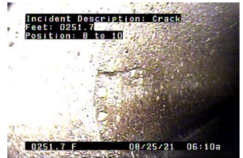
C - Crack @ 251.7 ft.
