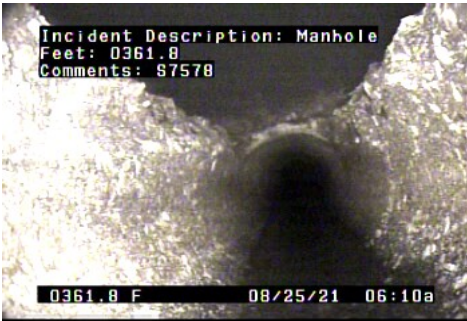
MH - Manhole @ 361.8 ft. S7578
