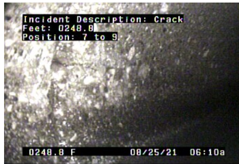
C - Crack @ 248.8 ft.
