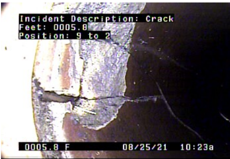
C - Crack @ 5.8 ft.
