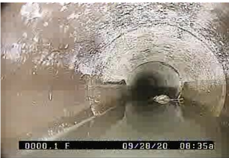
AP - Access Point - Other @ 0.1 ft. Manhole S3283
