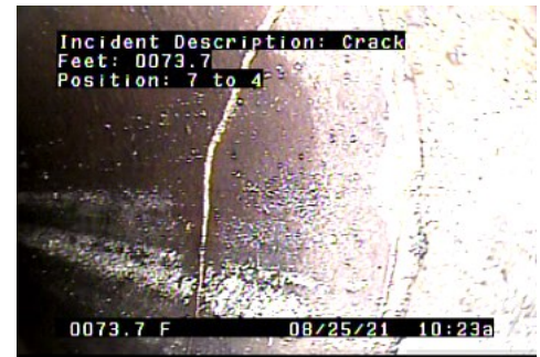
C - Crack @ 73.7 ft.
