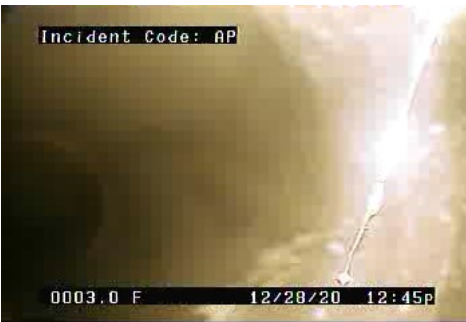
AP - Access Point - Other @ 3.0 ft. Manhole S6357
