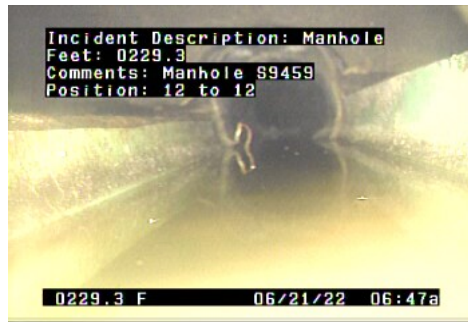
MH - Manhole @ 229.3 ft. Manhole S9459
