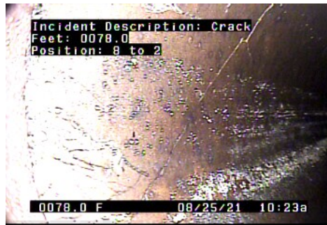
C - Crack @ 78.0 ft.
