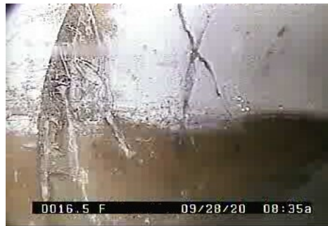
C - Crack @ 16.5 ft.
