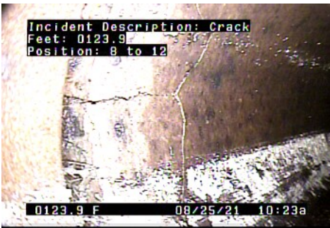
C - Crack @ 123.9 ft.
