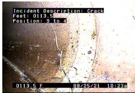
C - Crack @ 113.5 ft.
