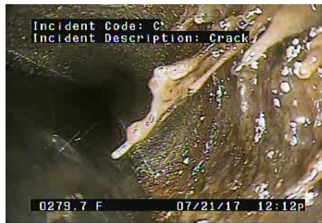
C - Crack @ 279.7 ft.
