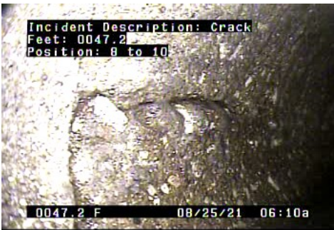
C - Crack @ 47.2 ft.
