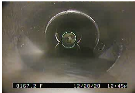
MH - Manhole @ 167.2 ft. Manhole S4048 ahead
