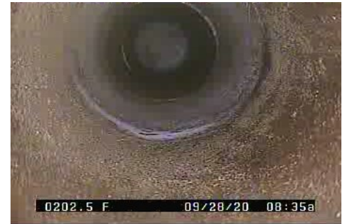
SC - Service Connection @ 202.5 ft. Not sure what this is?
