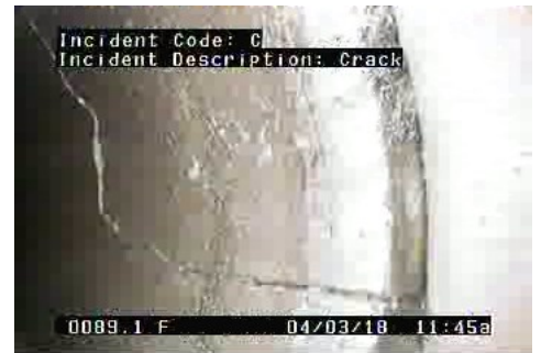
C - Crack @ 89.1 ft.
