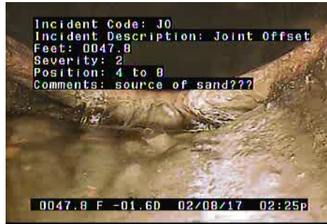
JO - Joint Offset @ 47.8 ft. source of sand???
