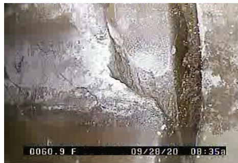
C - Crack @ 60.9 ft.
