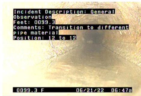
GO - General Observation @ 99.3 ft. Transition to different pipe material
