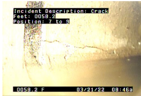
C - Crack @ 58.2 ft.
