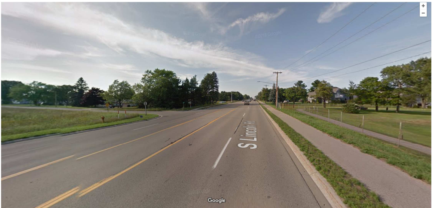
55. S Lincoln Ave and 14 th Ave S, looking north
