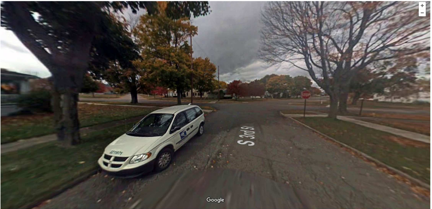
30. S 3 rd St and Ogden Ave S, looking north
